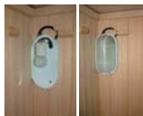
FIG-11 Assembling the light
