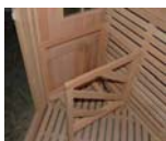
FIG-15 disassemble the wooden frame
